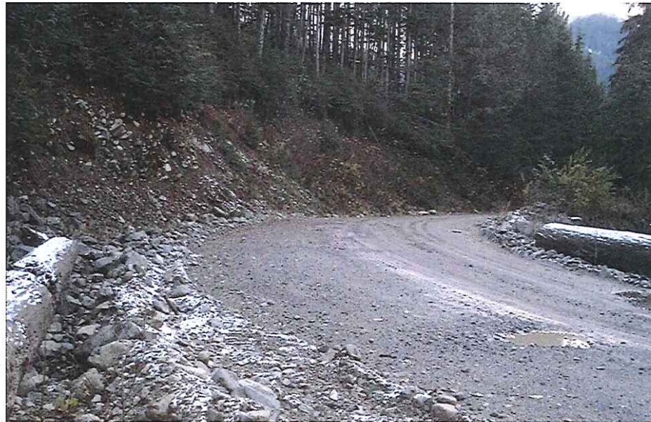
CK2454 Approach Right Bank
